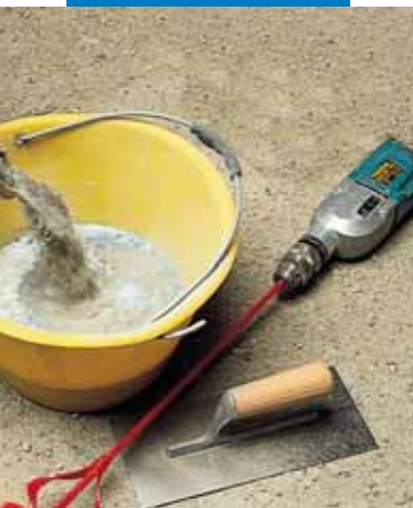
Mixing Mapelastic with a mechanical mixer
